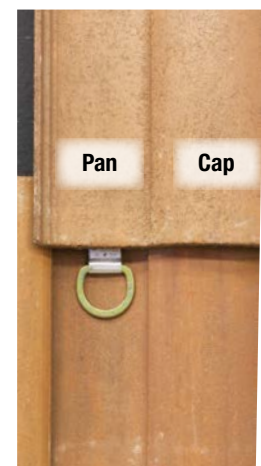
D-Ring exposure below Tile Head lap
