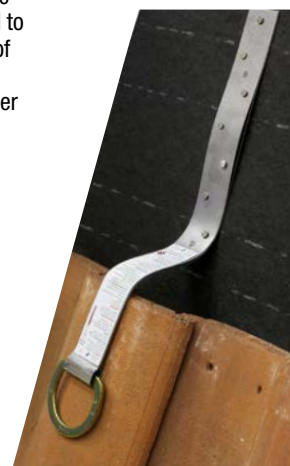
Plan D-Ring location and conform Anchor Leg to the tile profile.
