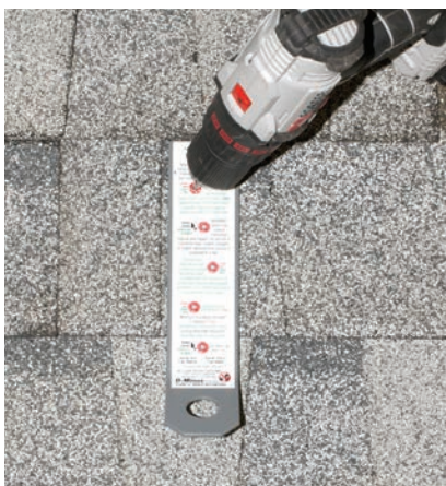
16) Attach anchor with SAS specified screws only.
