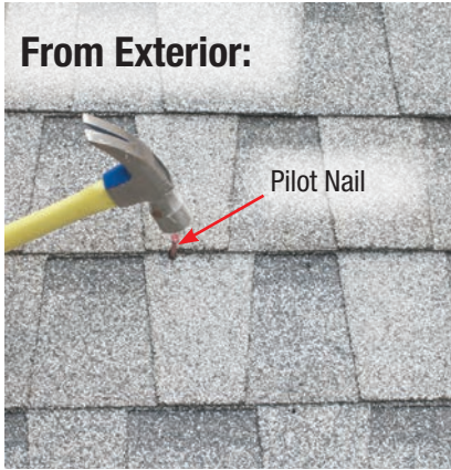
9) Plot anchor location and install a pilot nail.
