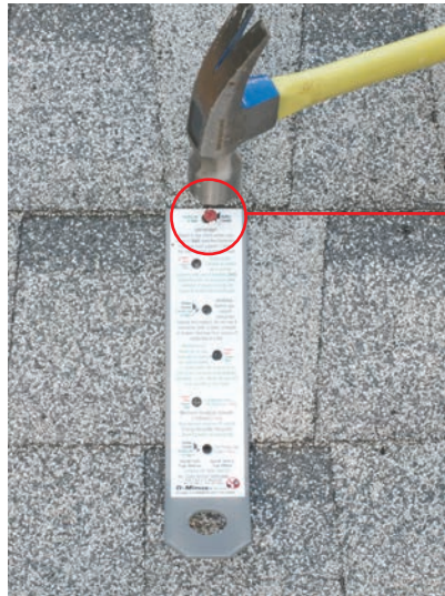
13) Position anchor and install a pilot nail through the anchor end.
