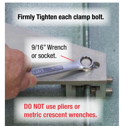
Fig.21 Clamp Bolt Attachment
