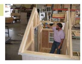
Install the 2x3 on the top of the door opening to strengthen the gable and fasten with 2 1/2" scews.
