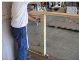
Fasten with 2 1/2" screws going from 2x6 into 4x4 on top.
