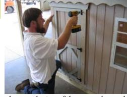
Install the door on the top of the spacer bar and center the door opening. Fasten hinges with 2 1/2" black heads.
