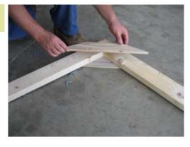
Use wooden gussets to tie rafters together and fasten with 1 1/4" screws.
