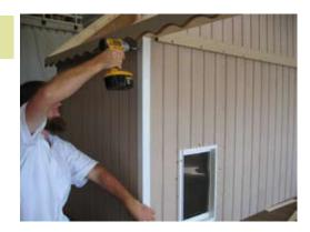
Install the aluminum corner trim and fasten with small white nails.
