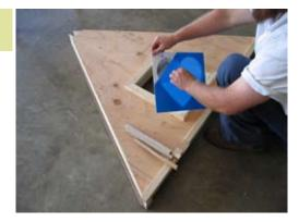
Measure 3" from the edge of the 2x6 to the edge of the rafter and fasten with 2 1/2: screw. This is for the dormer to set on.
