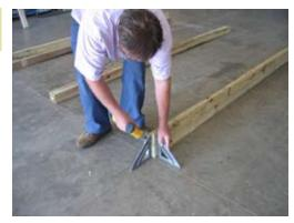
Fasten treated 2x4 rim with 2 1/2" screw into 4x4 runner use angle to make sure end and side is flush.
