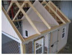
Also install (1) 2 1/2" screw from the bottom of the 2x6 into the rafter.
