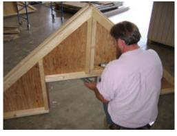
fasten the gable with 2 1/2" screws to tie together.
