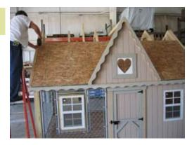
Install 2' OSB and fasten bottom corner with 1 1/4" screws.
