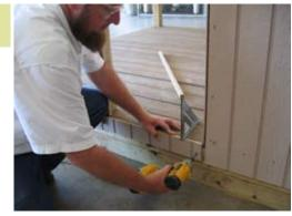
Install duratemp siding strip and fasten with 1 1/4" scews.
