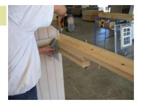
Use the angle and make sure the K-panel is flush on the inside of the 2x6 and fasten with 2 1/2" screws.
