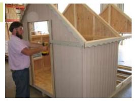
Install trim at the door and fasten with 2 1/2" screws.
