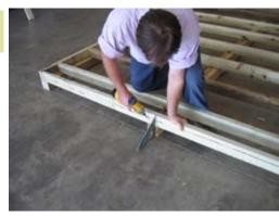
After the floor is square, fasten the joist to the center runner with 2 1/2" screws going in on an angle.
