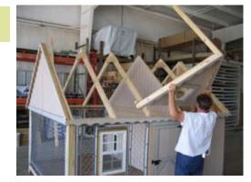
Top plates are marked off where trusses need to be placed.
