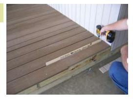
Use the floor spacer for gaps to install flooring until complete.
