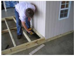
Next install the treated 2x4 to the side of the wall with 2 1/2" screws. This is where the flooring is going to rest.
