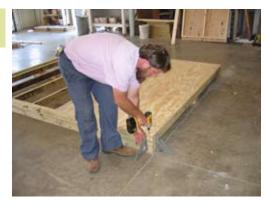
Install 4x8 CDX plywood. Use angles and make sure plywood is flush with 2x4 and fasten with 1 1/2" screws every 8".
