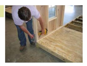
Locate the first wall panel and set in place. Make sure the wall is flush with the edge of the floor and fasten with 2 1/2" screws.
