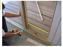
Make sure you have 20" from the siding to the 4x4 and fasten with 2 1/2" screws.
