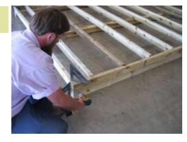
Fasten joist with 2 1/2" screws going thru the rim into the joist. Use angles to make sure all corners are flush.
