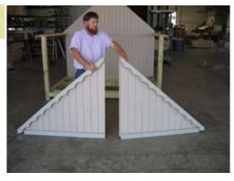
Next locate the gable for the opposite end where the gable is installed on the top of the 4x4 post.
