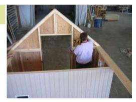
Use your angle and make sure the wall and the gable are flush and fasten with 2 1/2" screws.
