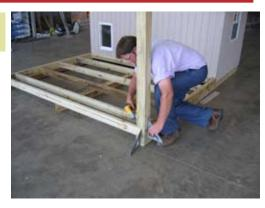
Next install 4x4 post and use angles to make flush with outside corners. Fasten with 2 1/2" screws on an angle.
