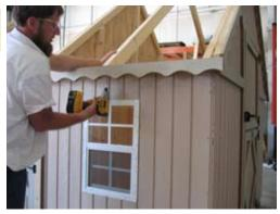
Installing rafters. Use angle and make sure it is flush with the edge of the 2x6 top plate. Fasten with 2 1/2" screw on each side from an angle.
