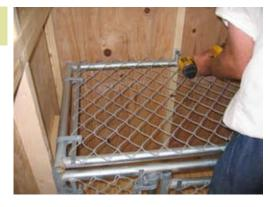
Next install the top panel as shown and fasten with screw and washer into 2x2.
