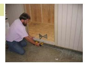
Install duratemp strip and fasten with 1 1/4" screws. Use angle to make sure it is flush with the floor.
