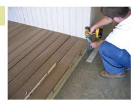
Use your angle where the notch is for the child door, to make sure it is flush and fasten with decking screws.
