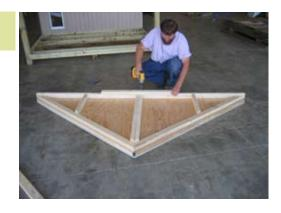
Install the 2x3 on the bottom of the gable end and fasten with 2 1/2" screws to strengthen the gable.
