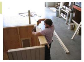
Install 2x6 top plate with trim as shown. Fasten with 2 1/2" screws every 16".
