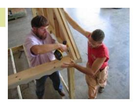
Install the gable as shown and fasten with 2 1/2" screws.
