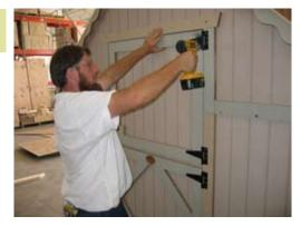
Install bottom door first and center door. Fasten with 2 1/2" black headed screws.
