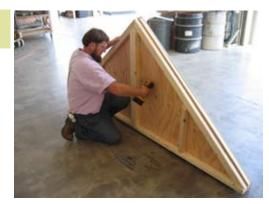
Secure the gable with 2 1/2" screws to tie the gable together.
