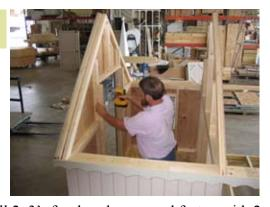
Install 2x3's for door braces and fasten with 2 1/2" screws.
