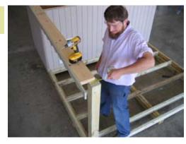
Measure 3" as shown to place top plate and fasten with 2 1/2" screws.
