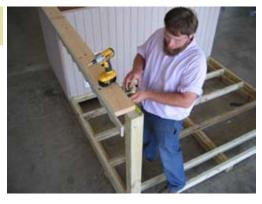
Measure 2 1/2" from the outside of the post to the top plate as shown and fasten with 2 1/2" screws.
