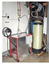
All wired for safety.. including GFCi protection Also.. ForkLiftable Skids are available, ..and standard on 20 to 50hp versions.
