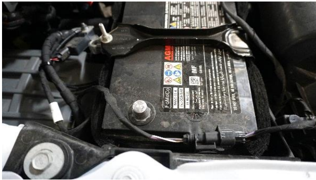
Primary Battery - Passenger Side
