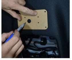
**4.** Use a sharp pick to create the holes for mounting the Keypad. Use a razor blade to cut the hole for the harness. Use the 5/32" and 3/4" bits respectively if mounting to a tougher surface.
