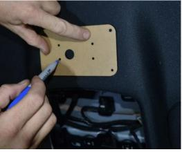
**4.** Use a sharp pick to create the holes for mounting the Keypad. Use a razor blade to cut the hole for the harness. Use the 5/32" and <sup>3</sup>/<sub>4</sub>" bits respectively if mounting to a tougher surface.
