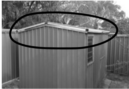
Oscillot® installed around shed roof perimeter to prevent cat from jumping on top of shed.
