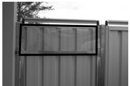
A gate with clear polycarbonate sheeting installed just below Oscillot® eliminating the horizontal rail so the cat cannot use it to get leverage.
