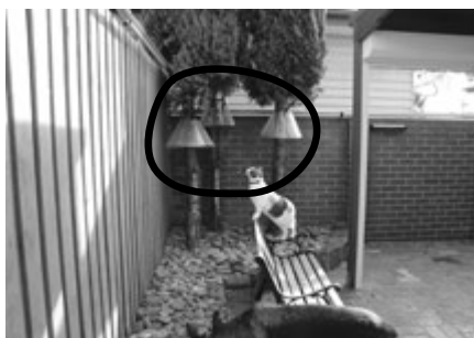
Oscillot® installation with tree guards preventing climbing up the trees in the corner.
