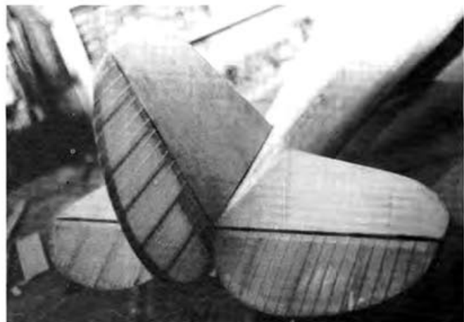
Complete tail installed. Controls are pull-pull cables. Elevator cables are inside vertical fin.
