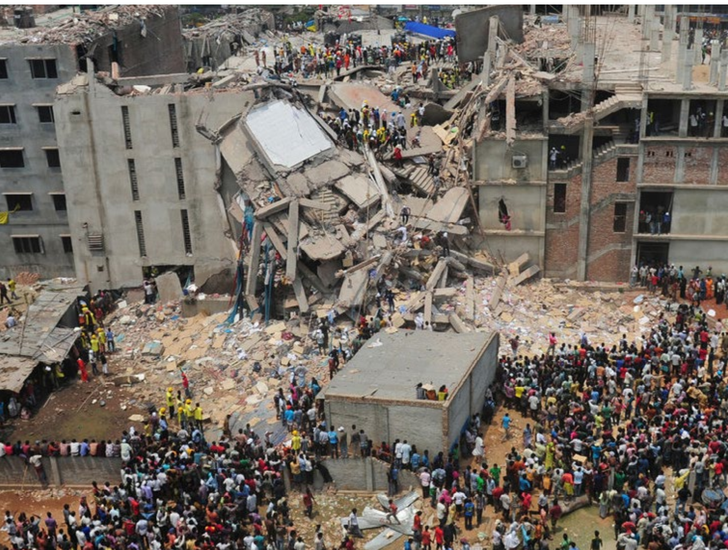
RANA PLAZA FACTORY COLLAPSE, BANGLADESH, APRIL 24, 2013
