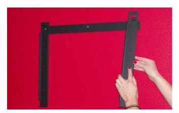
Replace the vertical brackets and using the anchor screws secure and tighten each vertical bracket to the wall. Your fireplace is now ready to be mounted.
