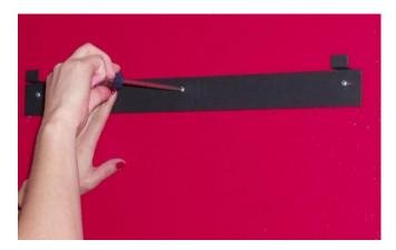
Place the horizontal bracket on the wall in line with the anchors and using the anchor screws secure and tighten the bracket to the wall. Hang the vertical brackets off each tab on the horizontal bracket. Using a level, level each side bracket and mark the holes.
