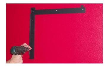
Line up the tabs on the horizontal mounting bracket with the two mounting cutouts located on the back of the backer. Lift the fireplace into position and make certain the tabs are locked into the mounting holes and the unit is seated securely on the wall. The tabs on the vertical bracket will sit under the backer.
