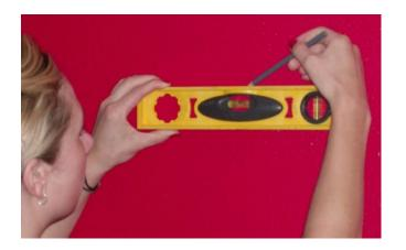
Take the horizontal mounting bracket piece (piece with tabs at top) and place it on the level line you drew. Mark the holes with a pencil and remove the bracket. Using a ¼" drill bit, drill the holes you just marked. Take the white plastic anchor and tap one into each drilled hole using a hammer. Make certain the anchor is flush with the wall.
