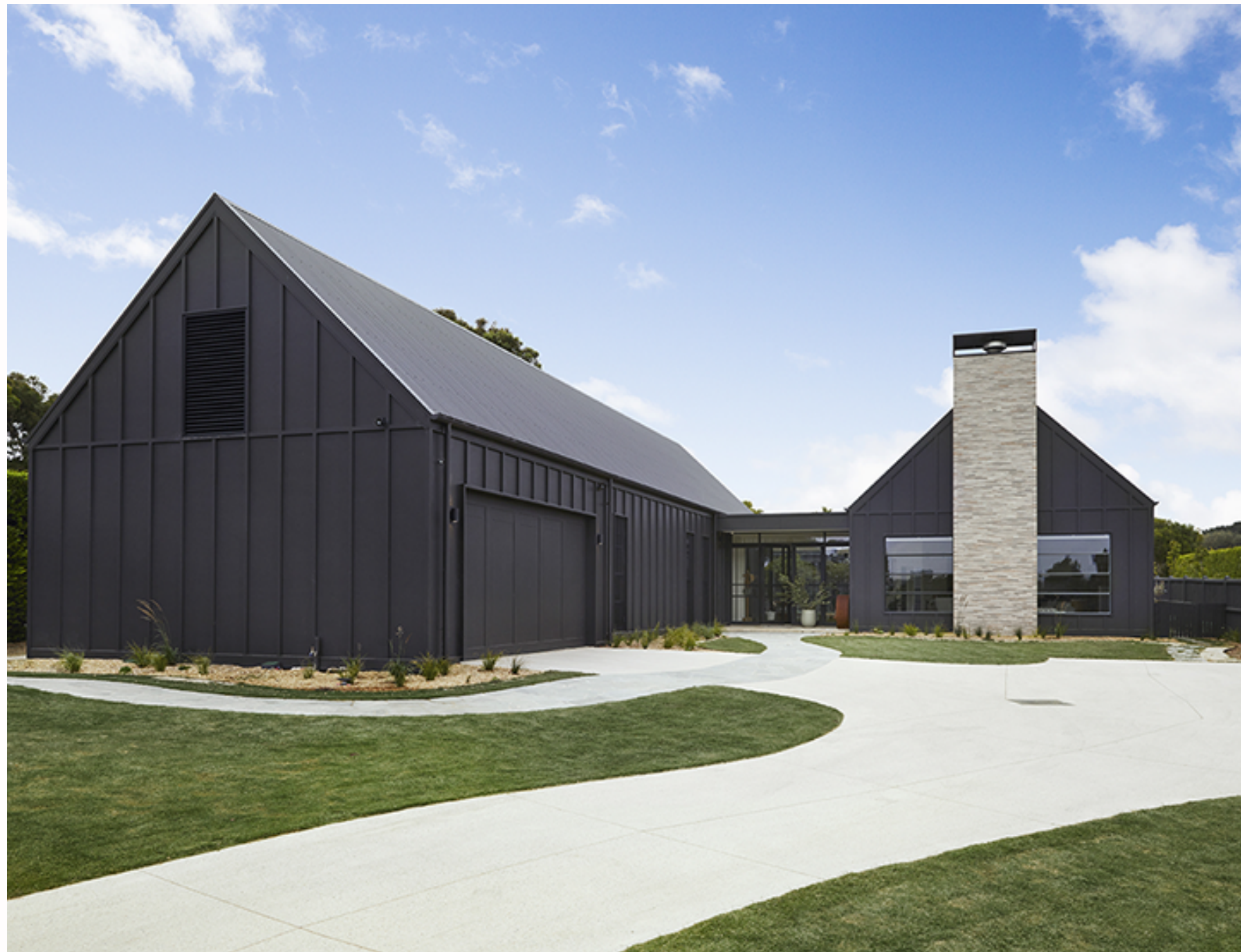
'Flinders' by Abe McCarthy Architects, Mornington Peninsula
