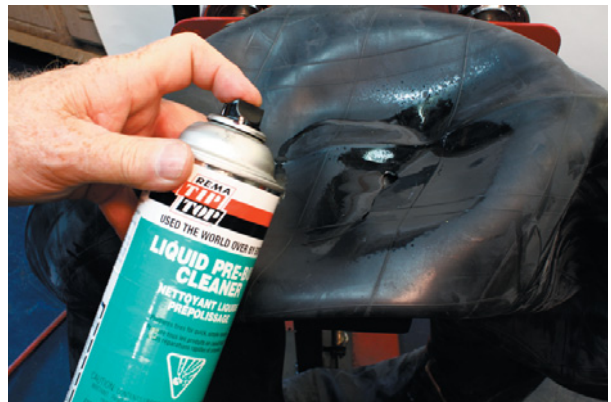
4. Spray Pre-Buff Cleaner to clean the repair area.
