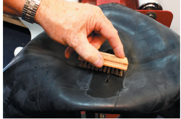
8. Clean the buffed area by using a brass brush.
