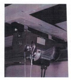
A typical ceiling installation with a 2x6 cribbed cross section securely fastened with 6, 3.5" framing screws.
