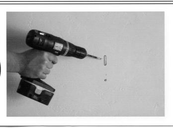
Using the metal frame as a template mark your holes in the center of the stud line.
