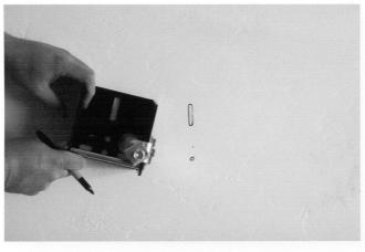
Using the metal frame as a template mark your holes in the center of the stud line.
