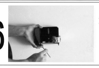
Attach the spool less metal frame to the wall using the supplied lag screws and washers. Center the frame before completely securing lag screws. Do not overtighten.
