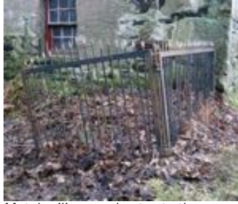
Metal railings and gates to the private gardens
