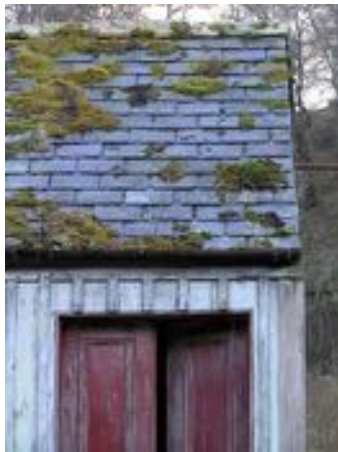
Detail of the shopfront
