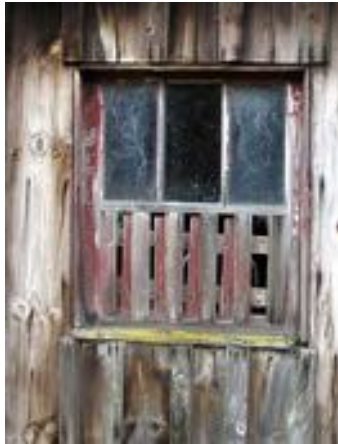
Detail of window and ventilator to the steading
