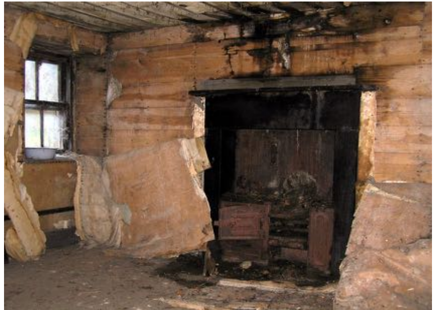
Boarded wall linings to the kitchen and cast-iron grate
