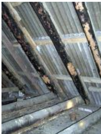
Interior of the roofspace showing half-rounded smoke-blackened timbers
