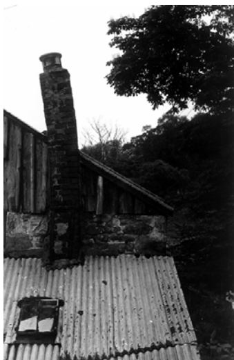
Former brick chimney to the wash house
