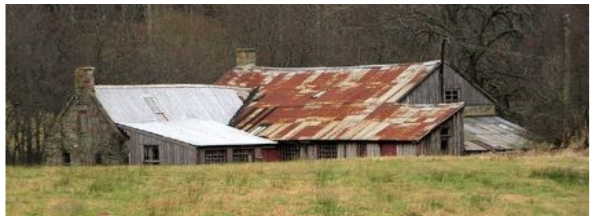
The mill from the southwest
