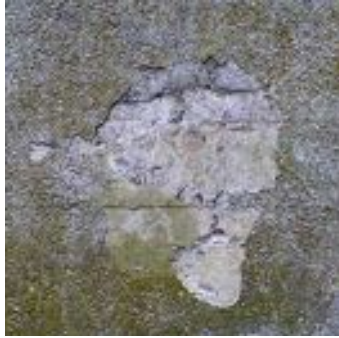
Detail of shuttered mass concrete wall to the weaving shed
