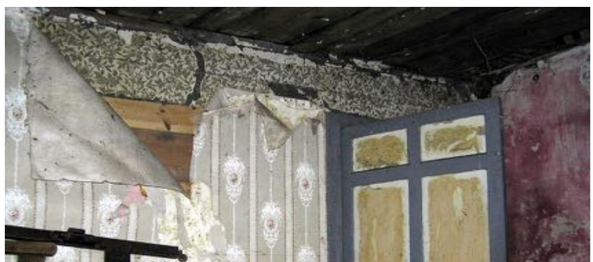
Layers of wallpaper to the living room
