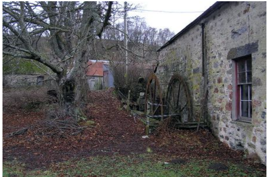
The waterwheel with the end of the penstock visible
