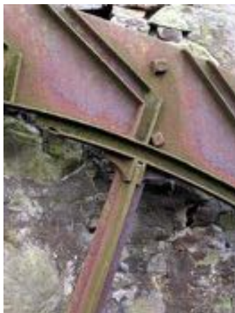
Detail of the waterwheel installed at Knockando
