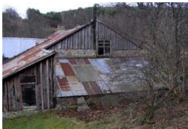
Southwest elevation of the mill shed
