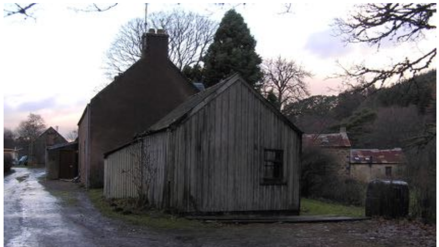
The shop gable on the approach to the mill
