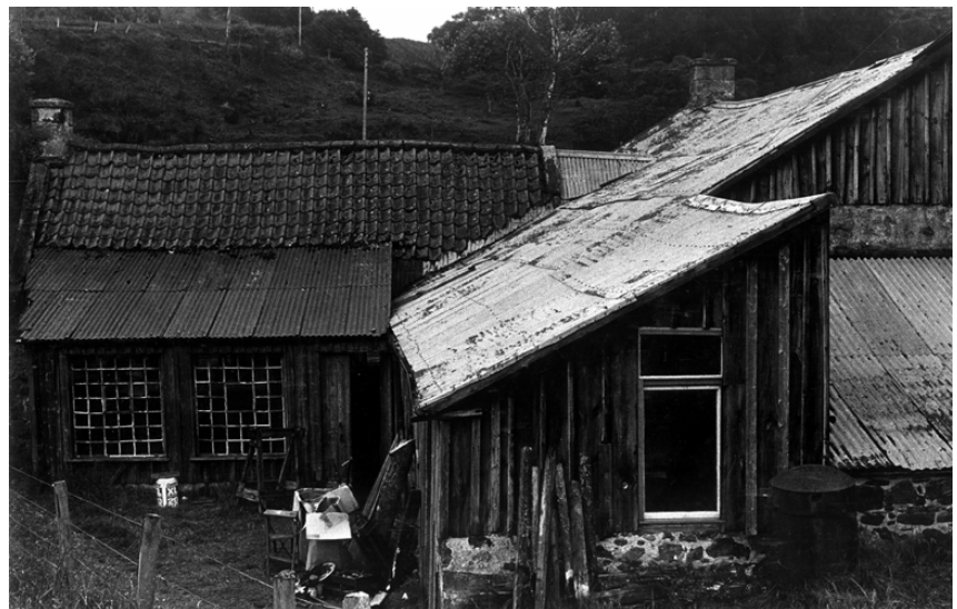
Photograph of the mill taken before the pantiled roof was removed (courtesy of Hugh Jones)
