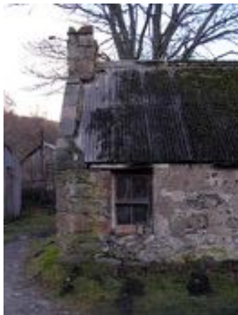
Window introduced to the kitchen
