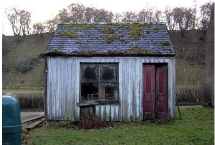
Elevation of the shop facing the former road
