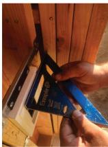
**5.** Check the thickness of drywall to be installed and adjust the SeeLess black perforated aluminum brackets, to either 1/2", 5/8", or 3/4" line (holes are perforated to the standard market perforation size)
