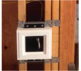
**4.** Verify studs are level by using a straightedge across the platform. Furr out each side, if necessary, so that the platform is leveled with the drywall.
