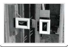
2 Screw thes two plates together: the Araknis metal backplate for dropped celling and the Araknis plastic mounting bracket.
