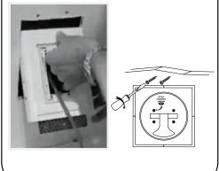
4 Level the drywall with the lower line of the joint on the front of the gypsum platform.
