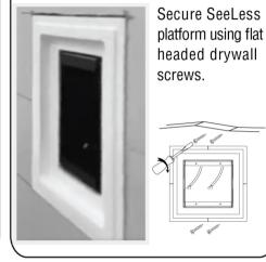
5 Cover the inside of the platform with paper or tape to protect the center opening. Apply the fiberglass tape on all four joints around the platform.
