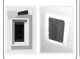
6 Sand surface smooth. Apply one coat of primer and wait for it to dry. Apply two coats of paint (it is recommended that you paint inside of the opening).
