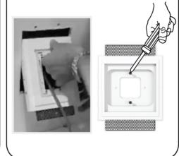
4 Level the drywall with the lower line of the joint on the front of the gypsum platform.
