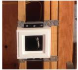
**4.** Verify studs are level by using a straightedge across the platform. Furr out each side, if necessary, so that the platform is leveled with the drywall.
