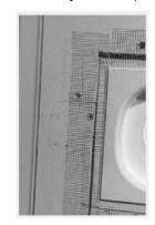
6 Sand surface smooth. Apply one coat of primer and wait for it to dry. Apply two coats of paint (it is recommended that you paint inside of the opening).
