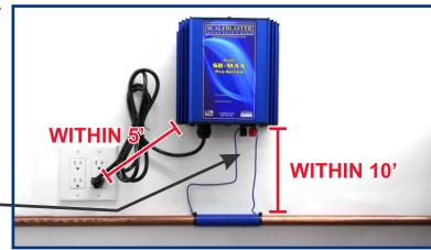
Install power unit in a well ventilated area.
