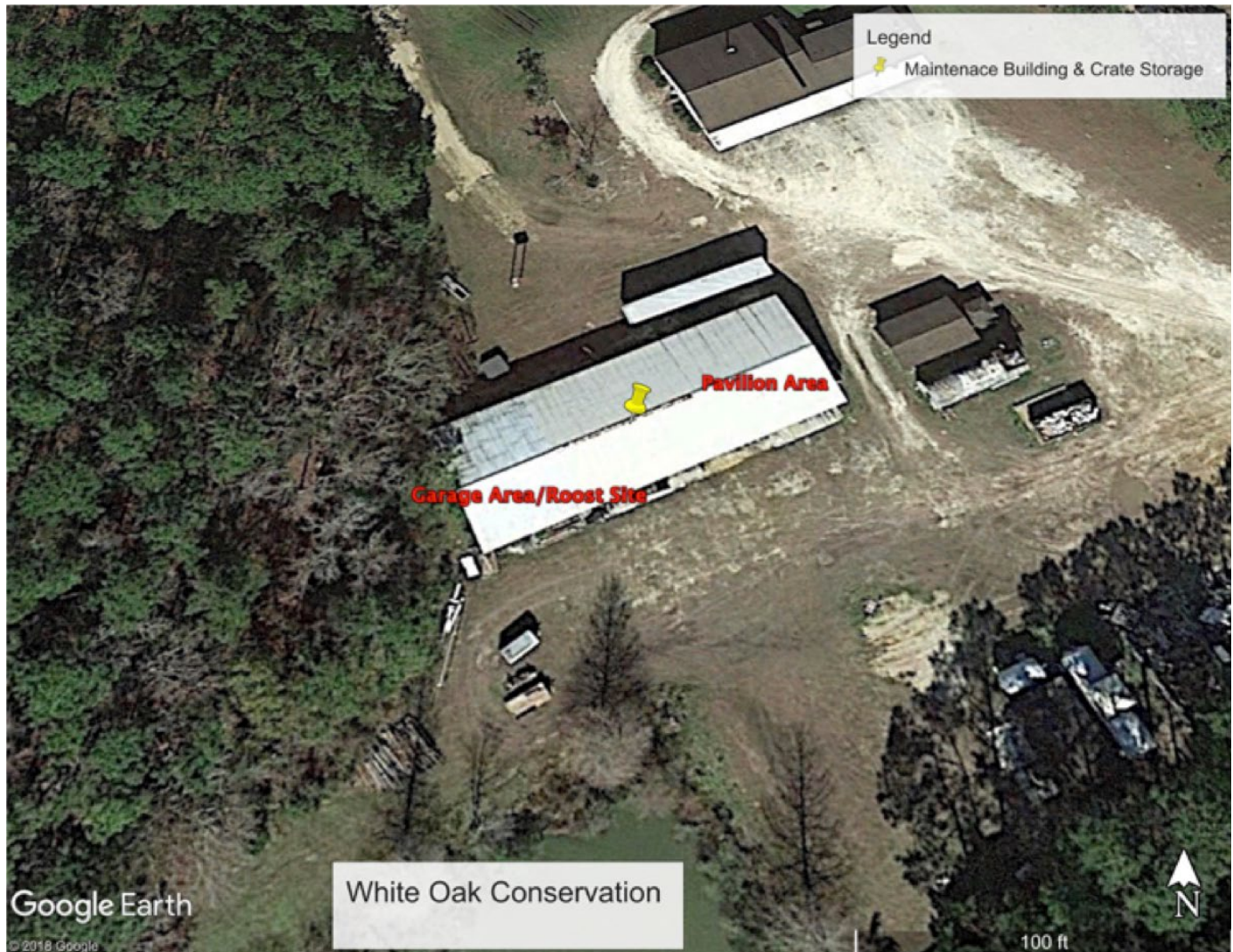
Figure 3-2: Bat roost site within the garage area of the maintenance building. This area is used for storage.
