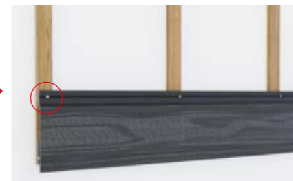
Pre-drill and screw cladding in place
