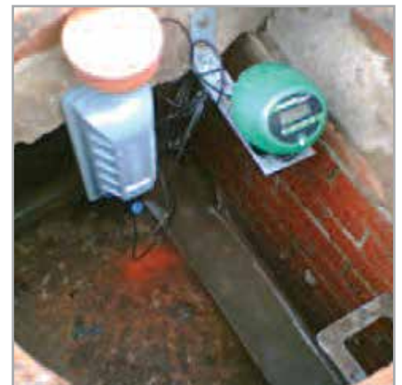
IMP Monitoring in a CSO Chamber
