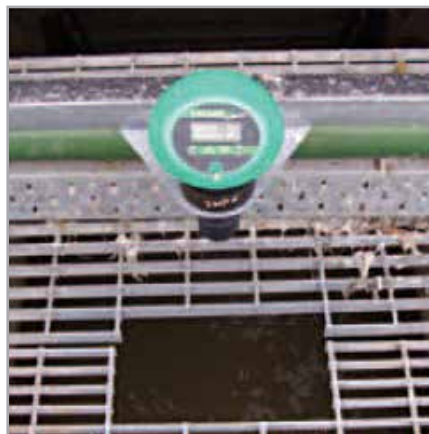
IMP Controlling Gate Height
