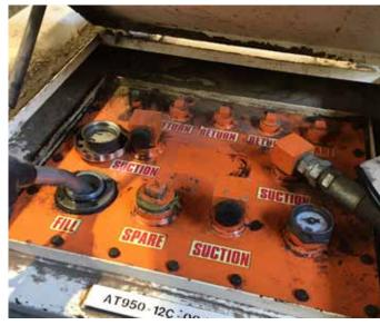
Be confident in the quality of fuel pumped into you machinery and equipment. The PETRO Technicians clean/drain your tank to ensure your fuel is clean, no water contamination and able to perform Polishing Fuel kits.
