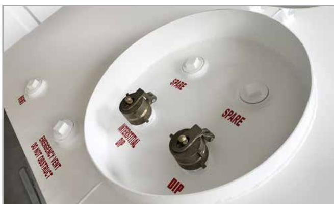
Dip and Interstitial Dip Points - enclosed in weatherproof housing
