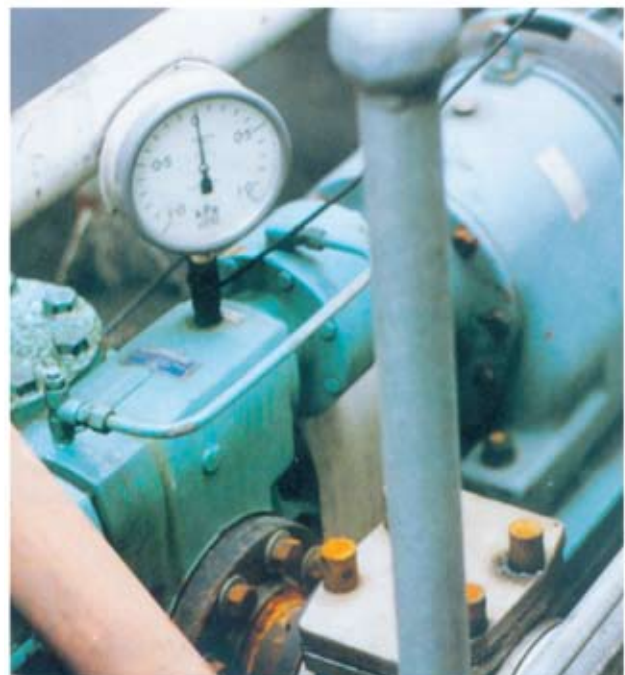
PFM Valve fitted to V40 Pump
