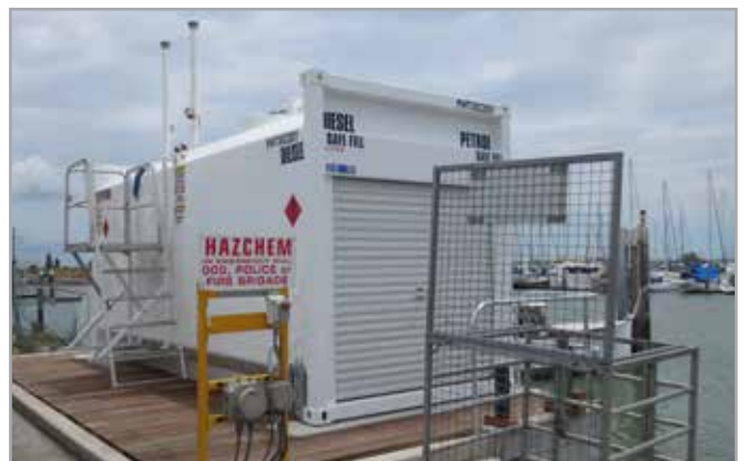
Diesel & Petrol Multi Compartment Tank
