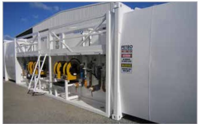
Multi Compartment Tank with Centre Pump Bay
