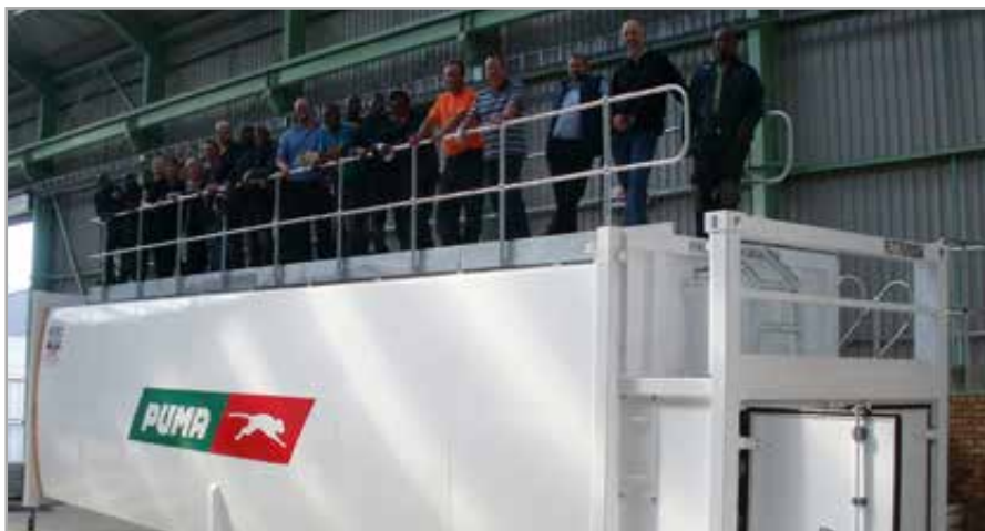
AS1657 designed and approved tank top access for dipping / maintenance of jiggle wire for floating suction / overall tank access
