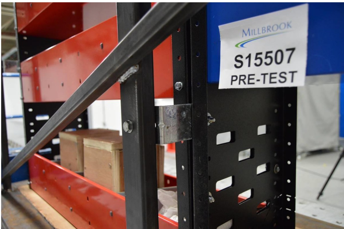
Close-up of StoreTidy/Standard-Heavy-Duty racking lower mount, pre-test
