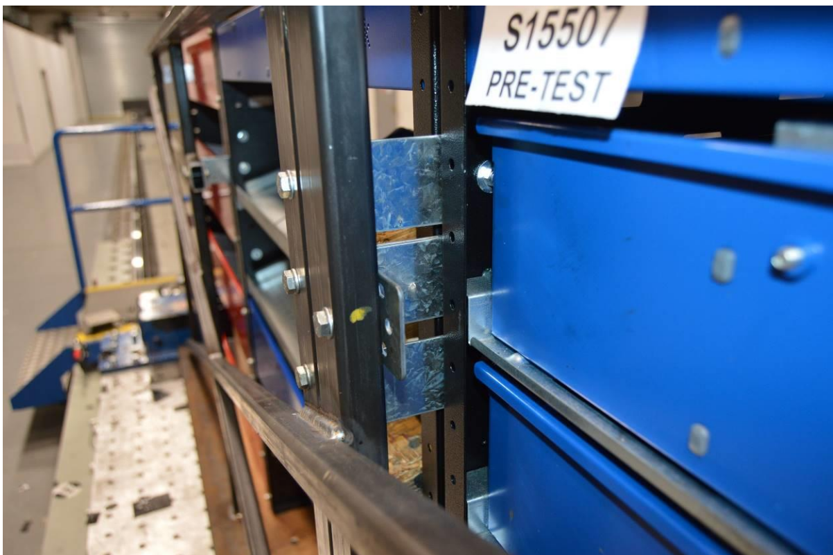
Close-up of Standard-Heavy-Duty/Extra-Heavy-Duty racking upper mounts, pre-test
