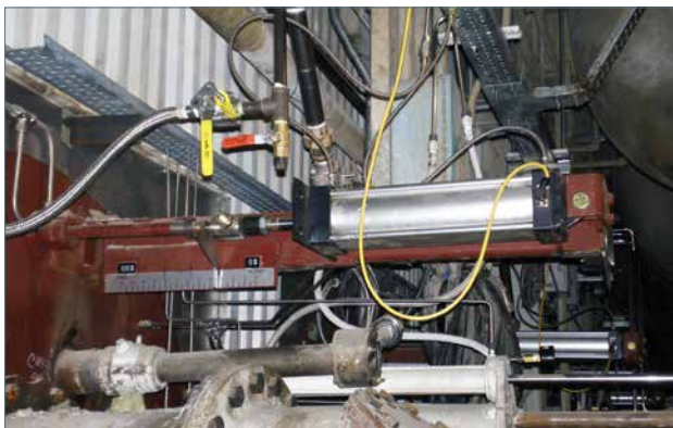
JR Series wall-fired burner shroud
