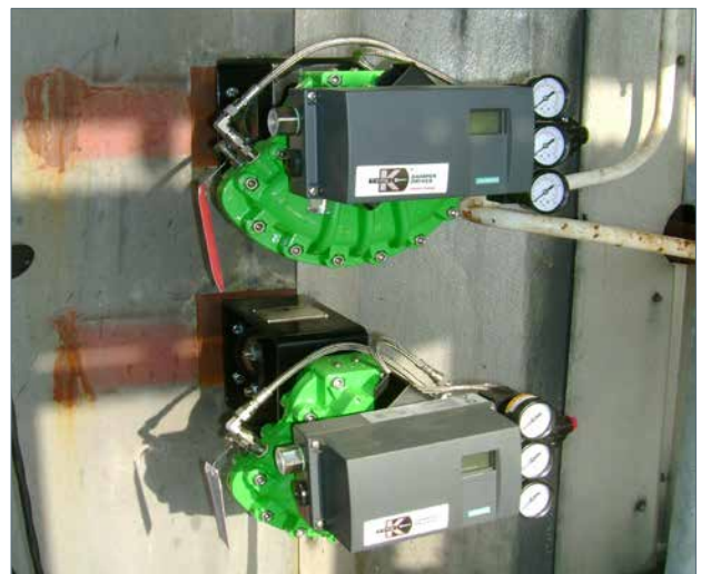
TYPE K DM Series on Windbox application
