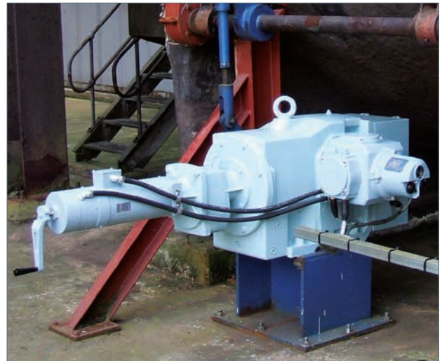
SM-6000 Series on Induced Air Fan Damper
