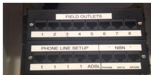
Around your home will be installed field outlet wall plates as per the sample to the right. These wall plates will all be numbered with the corresponding number that shows in the Smart Hub (on the harmonica)
