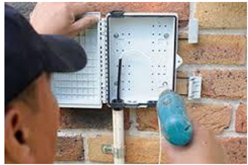
Network Termination Device installation
