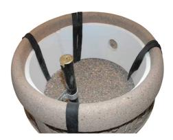
Pull wicks through the precut holes in the membrane. Place membrane neatly over the stone.
