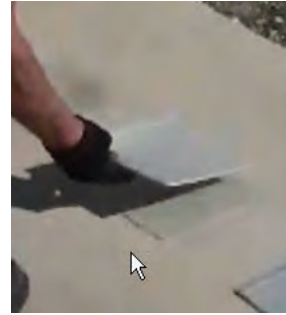
Placing Second Pad
