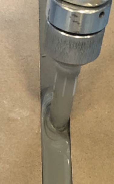
Application with Mapeflex SPP pump
