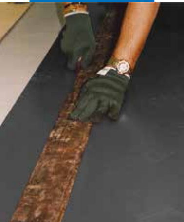
Cutting the joint between sheets of Mapelay
