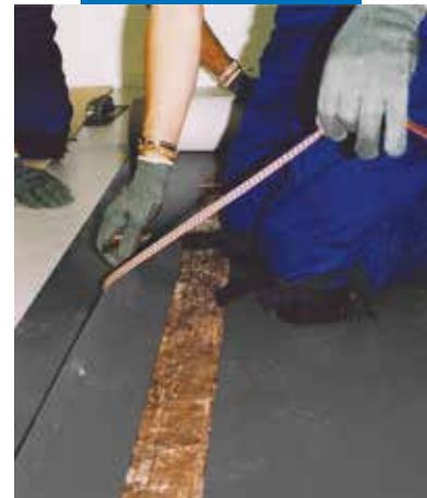
Removal of the cutted portion of Mapelay
