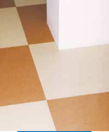
Tiled floor laid on Mapelay
