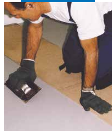
Smoothing the floor; avoid imprints by kneeling on a rigid panel
