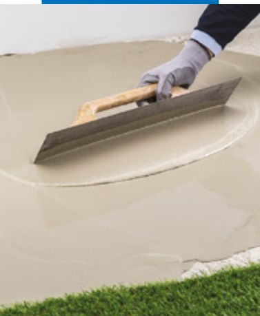
External application of Planex HR Maxi
