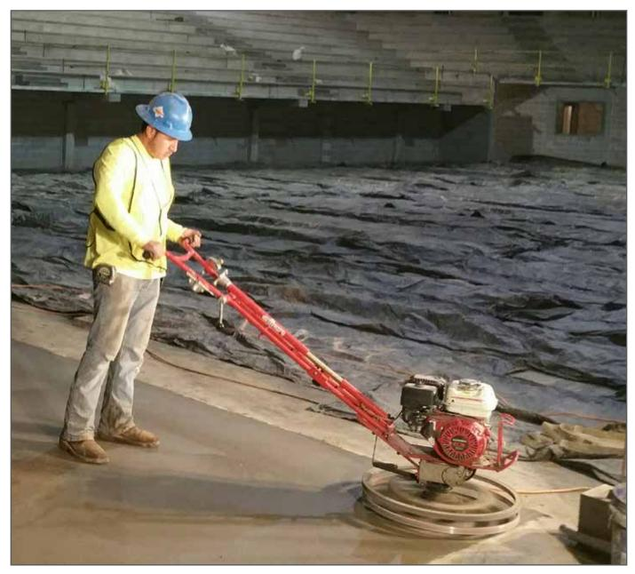
Allen Pro-Series Walkers feature precision engineered gearboxes for long, trouble-free life. We use cast iron spiders, pressure plates and lift levers for long wear and continuous service, and we precision machine our trowel arms and spiders to such close tolerances that our trowels do not requre bushings.
