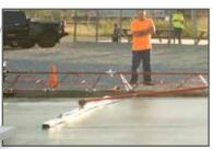
**CHECK ROD** Reduces bumps and fills low areas while the concrete is still plastic.
