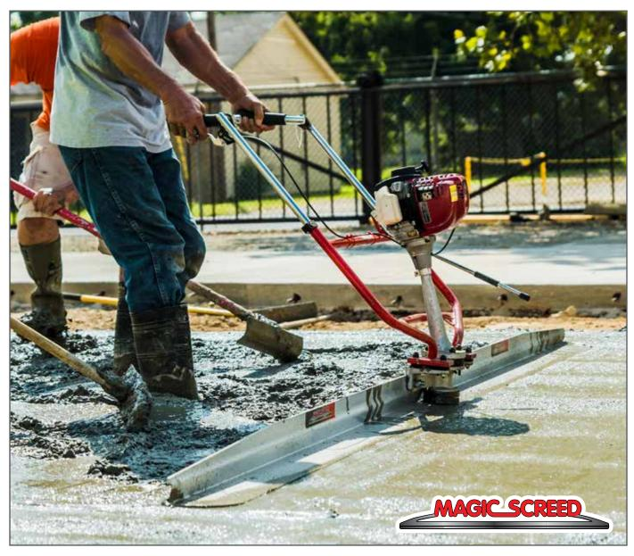
The Magic Screed is a precision engineered, lightweight wet screed for single operator strike-off of concrete. Fast and easy to use, this high-frequency screed provides uniform distribution over the entire blade length, enhancing structural integrity of the concrete through consolidation.
