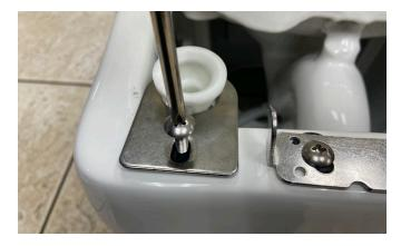
• Use a phillips screw driver to tighten back the screw holding the metal plate and the new cup.
