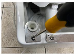
• Use a phillips screwdriver to take out the screw holding the cup.
