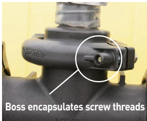
Tab protrusion is a safety hazard
