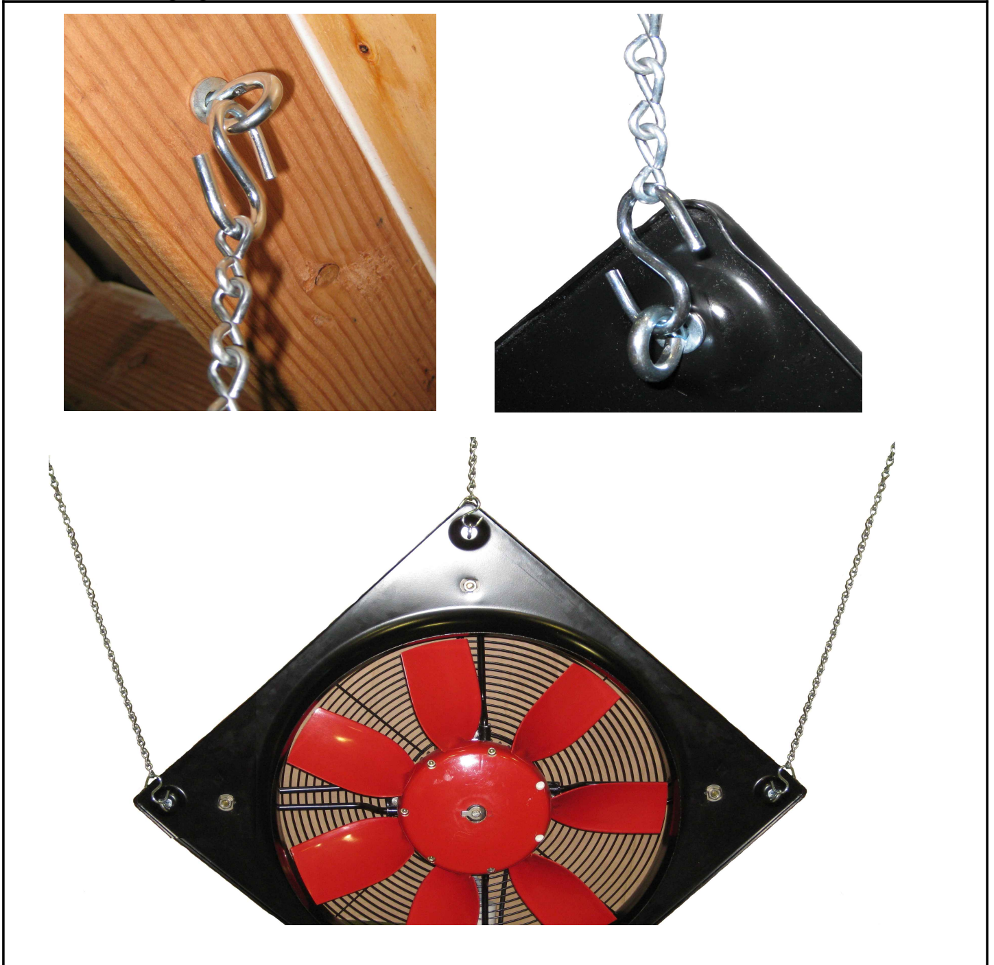
FIGURE 6– Hanging the Fan
