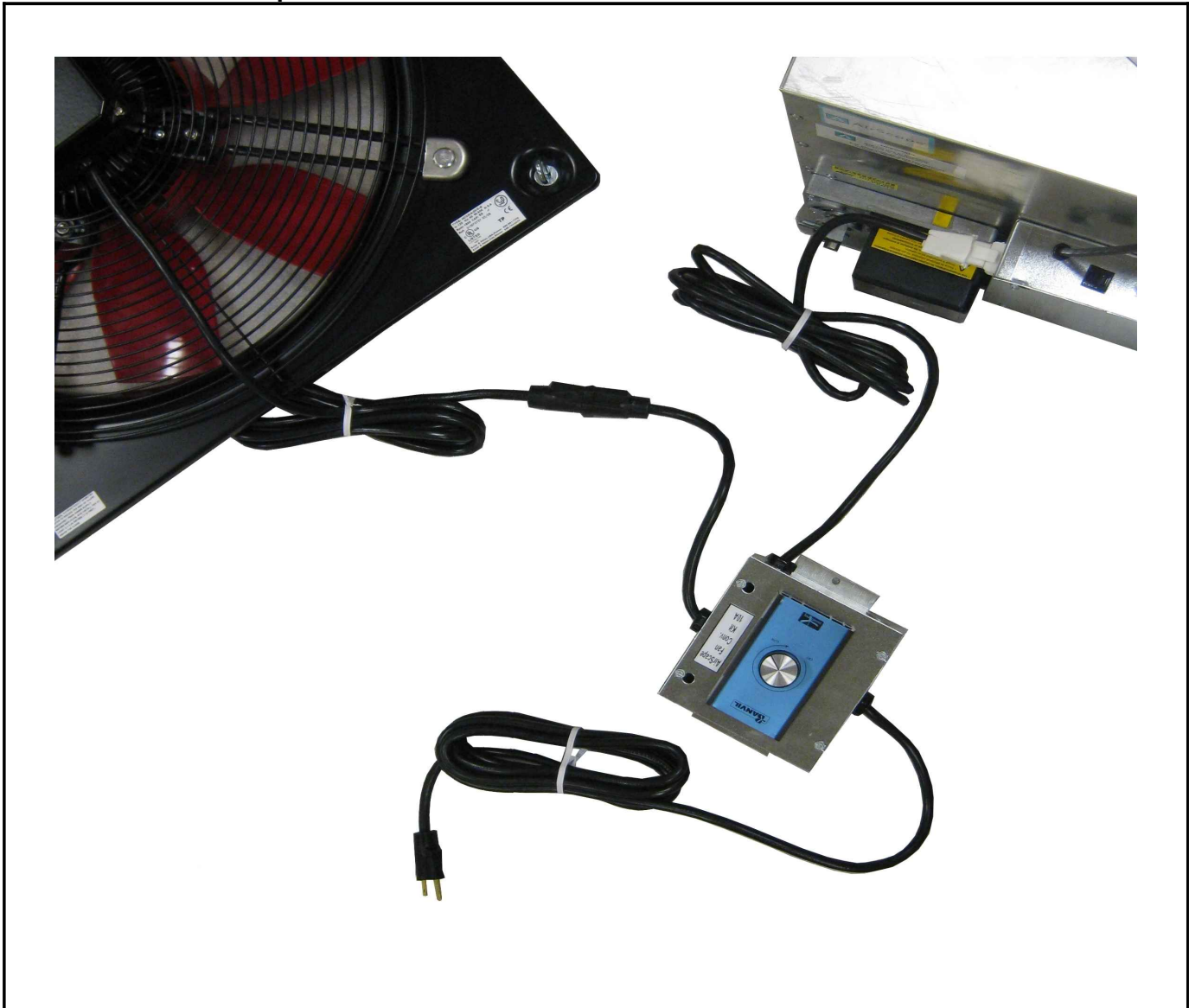
FIGURE 9 – Low Speed controller Installed
