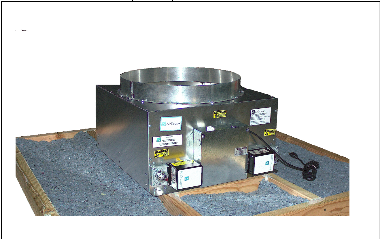
FIGURE 4 – 2.5 WHF Installed (attic view)
