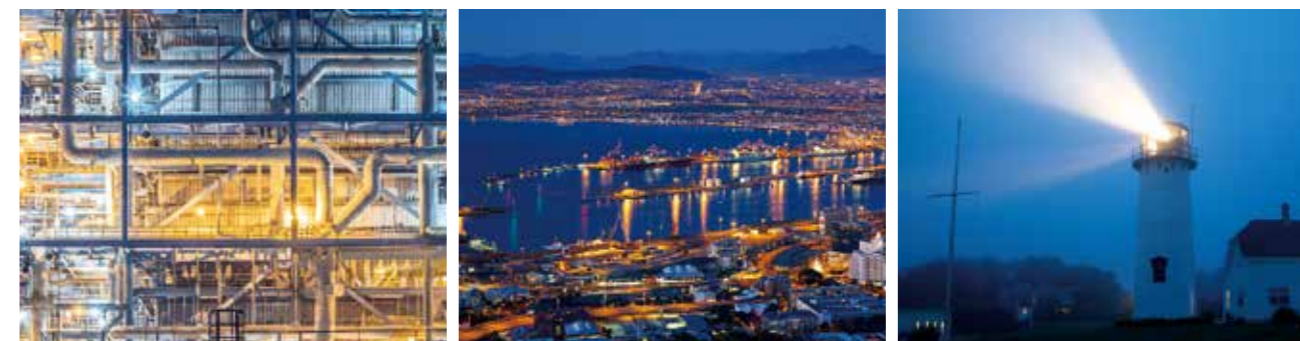
Public engineering area of chemical industry area
