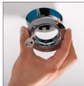
3. The downlight can now be safely and securely installed.
