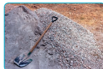
Mixing sand and gravel
